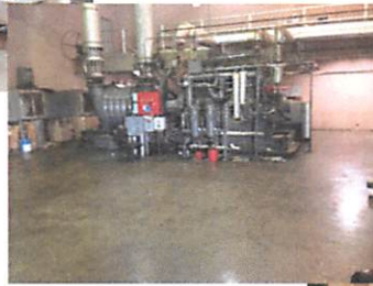
Engine and Blower with control panel
