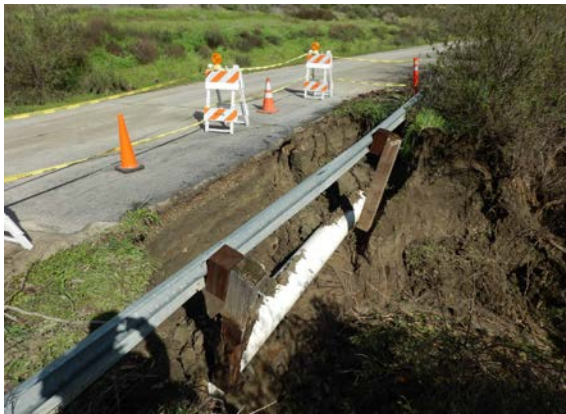
Erosion at Site West 1 (W1)
