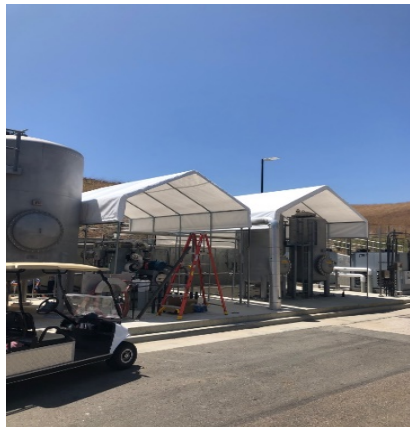
Shades were installed over the new gas skids to prevent overheating.
