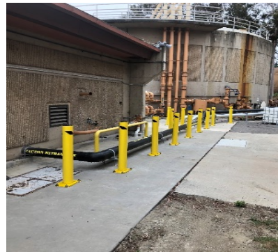
Ballards were installed to protect temporary digester gas pipe.
