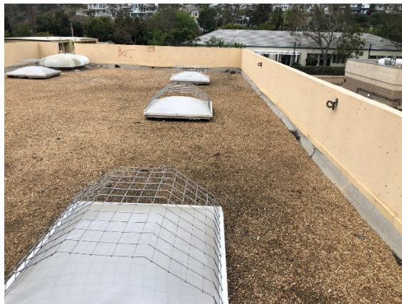
New skylights were installed at JBL that include fall protection Screens over the skylights.
