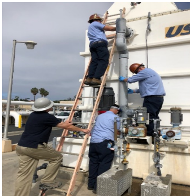
Staff replaced a recirculation pump at JBL, the Director of Engineering also lent a helping hand.
