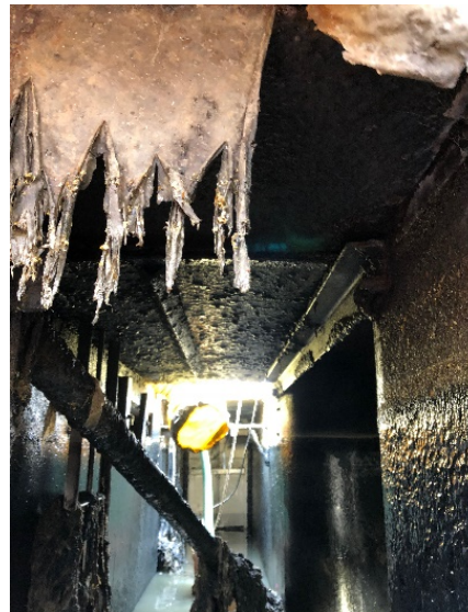
This is the Primary Influent Channel; the coating in the influent channel has completely failed. The channel needs to be relined near Primary Tanks #4 thru #6. The abandoned and collapsed pipe in the photo was removed.
