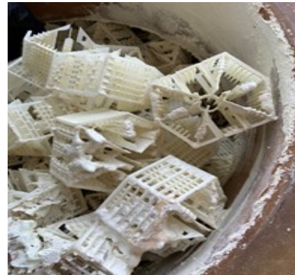
Media was replaced at CTP. This picture shows the buildup of calcium on the media over the past ten years that blocks the scrubber effectiveness over time.
