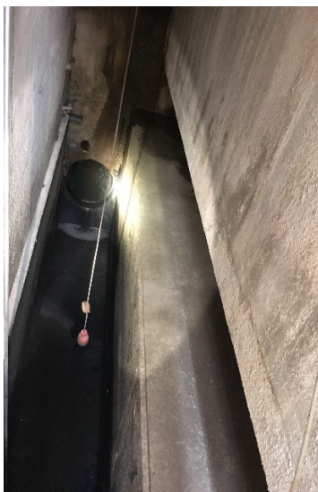
This is the wetwell for the influent pumps. The coating system needs some spot repairs near the influent pipe.
