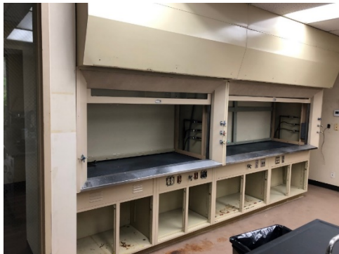
Asbestos removed from fume-hoods At CTP (by contractor).
