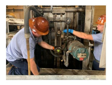
Pictured below, staff removed some large rocks and repaired the equipment damaged from the large rocks. The picture below is a damaged check valve.
