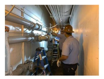
Shown below is a drier system installed by Staff on the polymer vent lines to prevent moisture from entering the tanks and creating unpumpable balls (aka fish eyes) of the polymer.
