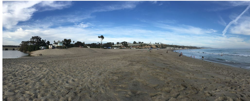
Buried Junction Structure – Current Condition
