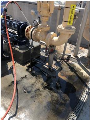
O&M staff regularly change oil and grease pumping equipment in the plants. Below are some photos of the equipment being maintained. Typical activities include draining and replacing oil, greasing bearings and motors, and inspecting drained oil. When O&M staff finds metal shavings, or other debris, in the drained oil that could impact the life of the equipment, they schedule the equipment for further investigation and assessment.
