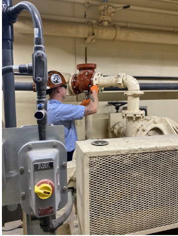
Grit Check Valves at RTP Replacement
