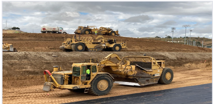
Wheel Tractor-Scraper removing soil on site
