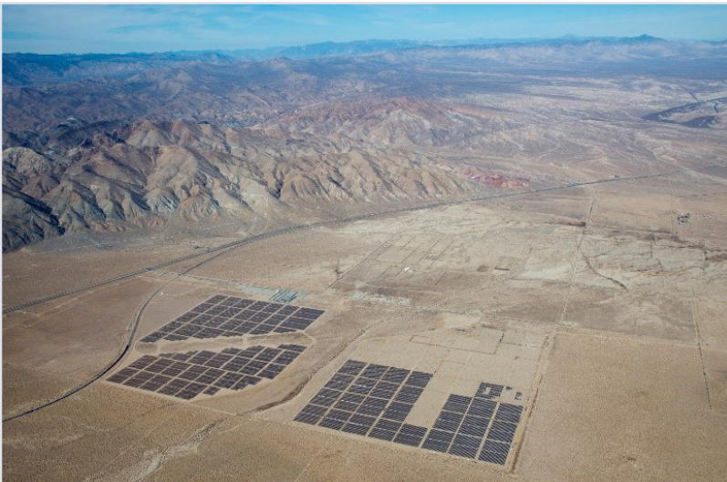
Beacon Photovoltaic project solar panels
