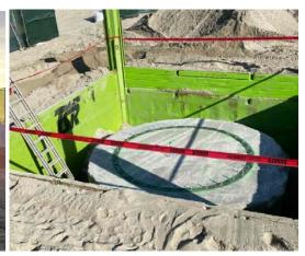
The contractor, Filanc, built a mock-up of the structure and sleeve pieces so divers could practice before entering the actual structure.
