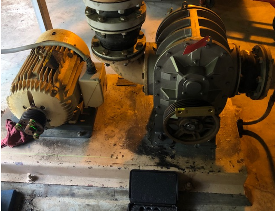
Low-pressure blower replacement and laser belt alignment.
