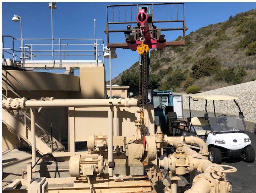
Daft recirculation pump replacement project.
