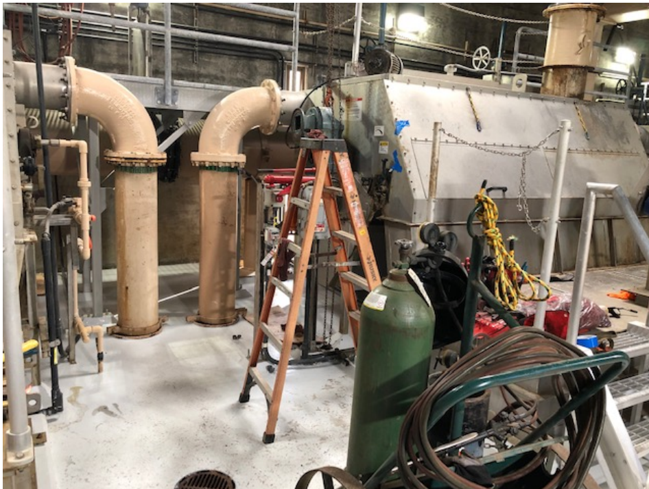
Center roto screen bearing and gearbox replacement.
