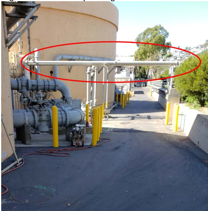
Digester 1 & 2 with Pipe Bridge
