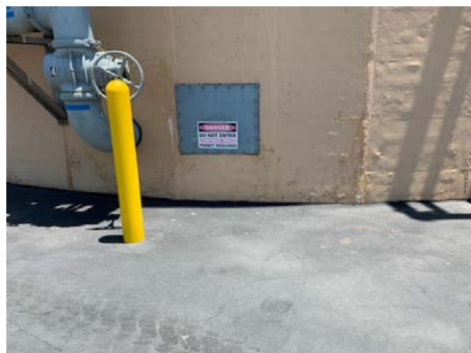
Existing Digester 2 Manway
