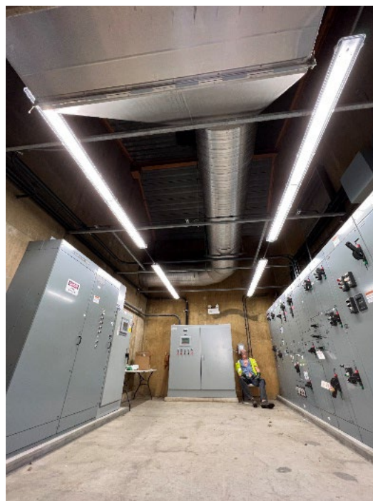
Staff replaced the obsolete and failing lighting system in the RTP Blower Room. (Before is on the left and after is on the right.)
