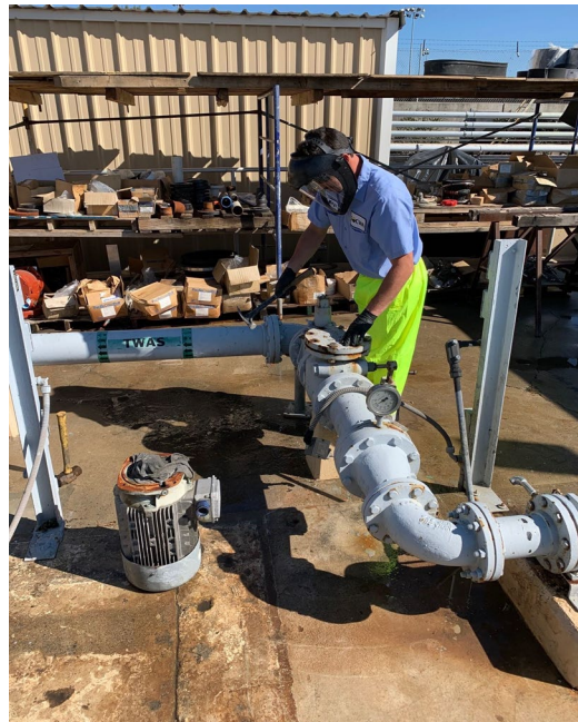
Failed TWAS check valve replacement at JBL.
