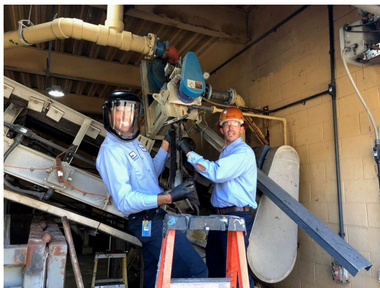
Repaired the seized rollers on JBL 9-Side Conveyor.
