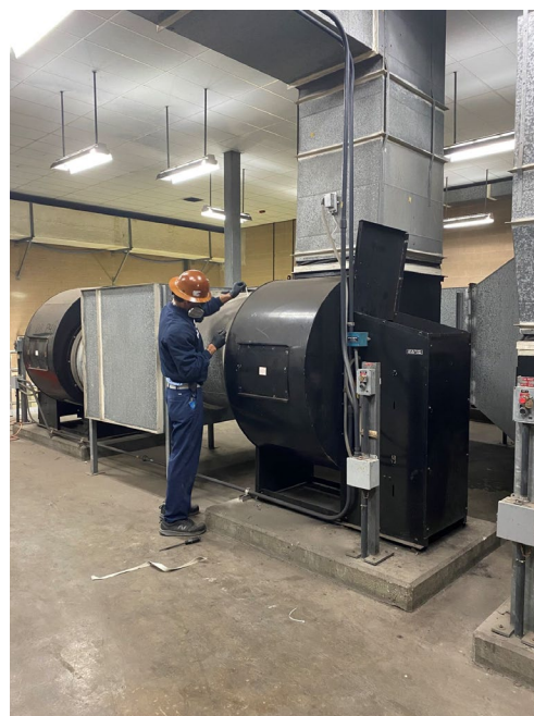
Replaced failed fresh air fan for Building 40 at JBL.
