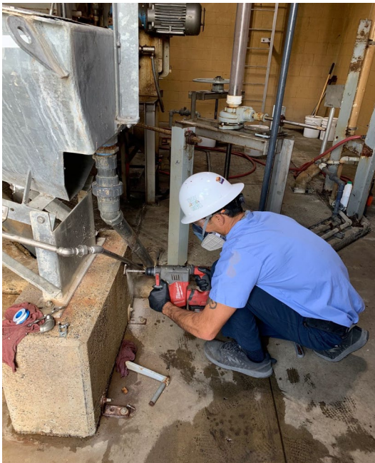
Grit Auger PVC flush line replacement at JBL.
