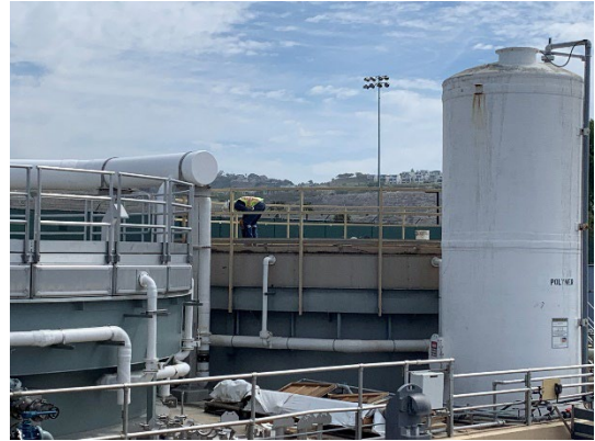
DAFT#1 demolition started
