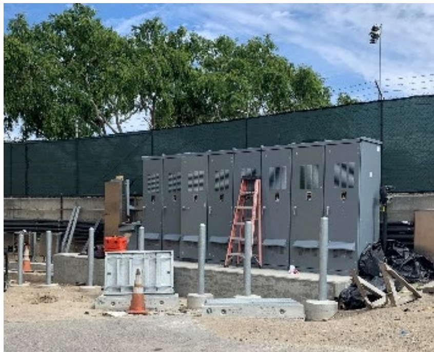
Newly energized MCC-F1
