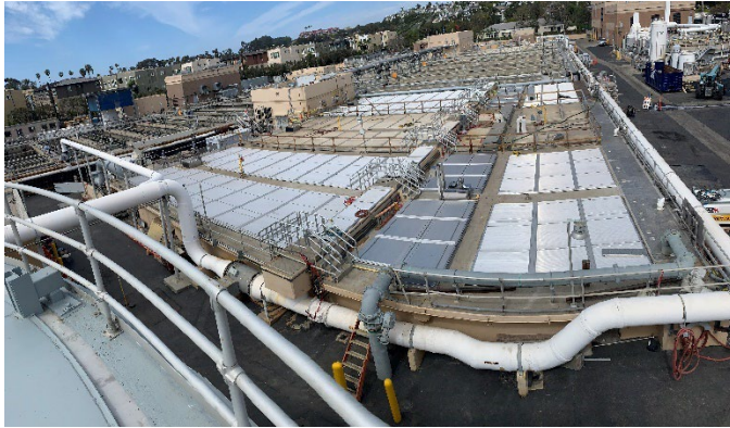
Completed Primary Basins Nos. 1 and 2
