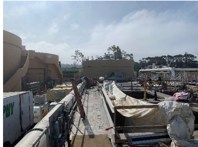
Completed Primary 3/4 Effluent Channel Covered and in Service
