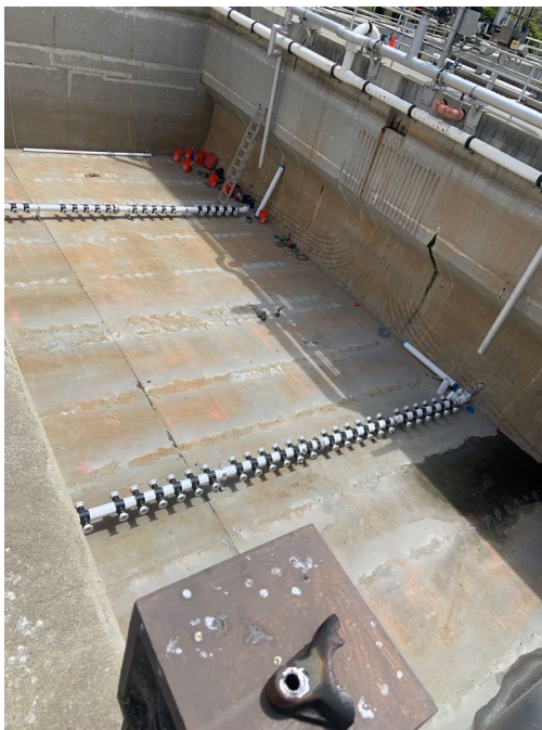
Starting Tank Work
