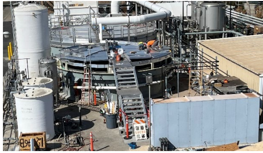
DAFT Cover Installation
