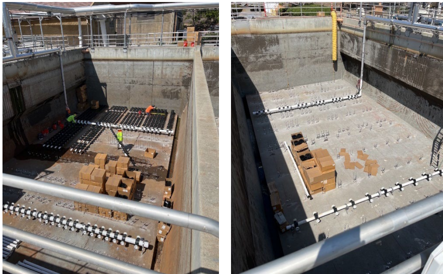
Diffuser Installation in Final Aeration Basin
