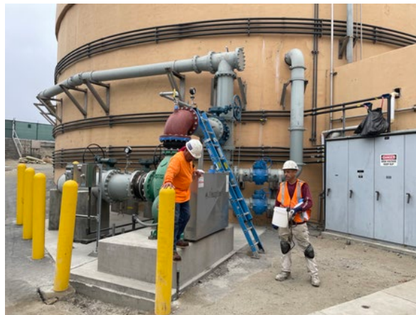
Installed Digester 2 Mixing Pump
