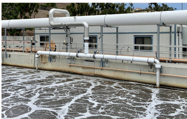
Aeration basin operating with new diffusers and new air header
