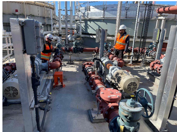
New TWAS Pump Station
