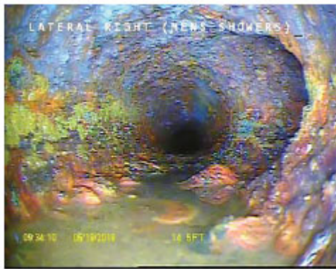
Lateral from the Right at 14.50 Ft.
