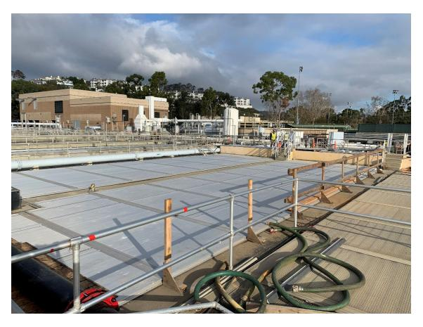
DAFT #2 has nearly all the mechanical equipment and piping installed. The electrical work is underway and anticipated to be complete in February 2021 for the DAFT #2 start-up.
