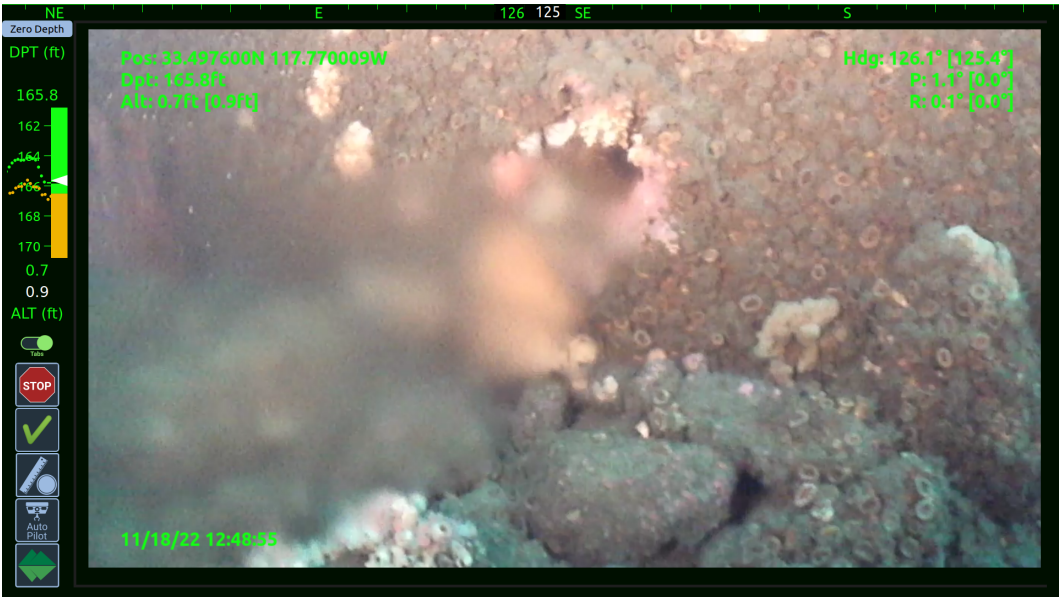
Photo 6 – View of an additional ACOO diffuser port, with effluent flowing
