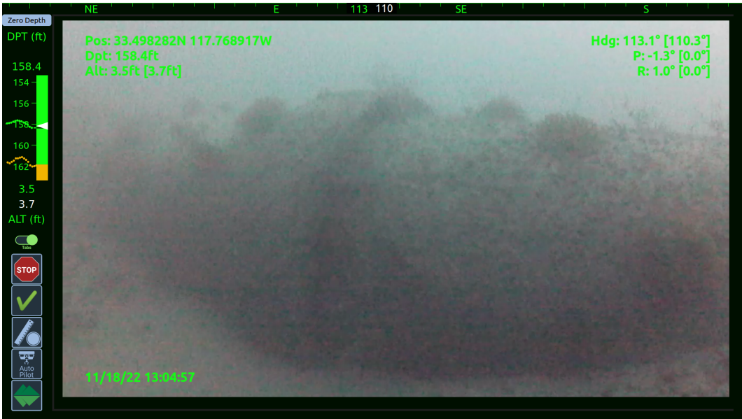
Photo 10 – View of an area along the ACOO that is missing ballast, well below the springline
