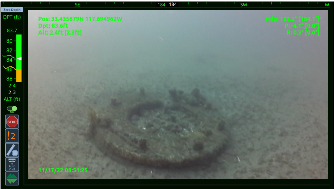
Photo 8 – View of an SJCOO outfall manhole, slightly protruding from beneath the sand
