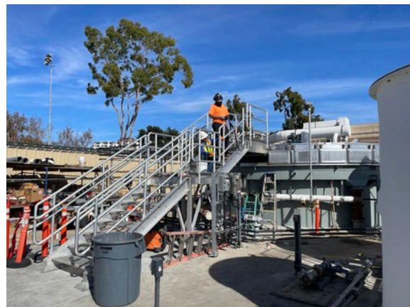
DAFT 1 Access Stair with Handrails
