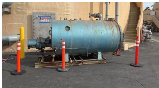
Old Boiler Removed from Digester Control Building
