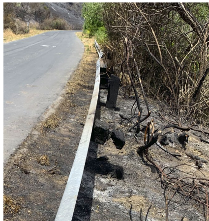
Figure 1: Fire Damaged Guardrail
