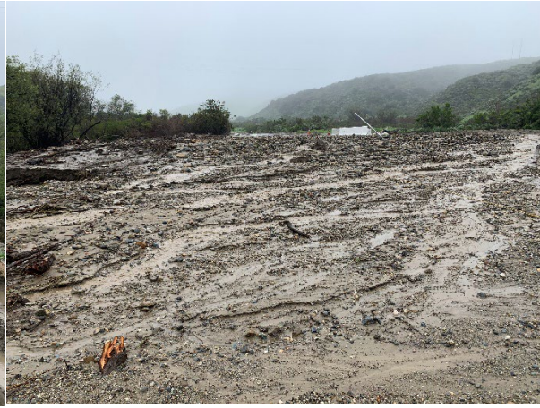
Photo 2: Buried East Access Road/Trail
