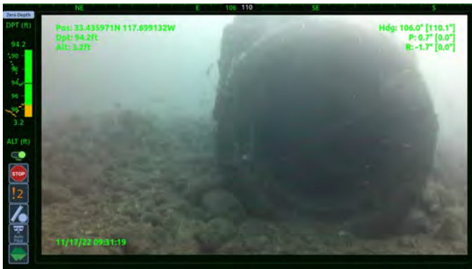
Entry 67 - End Structure
