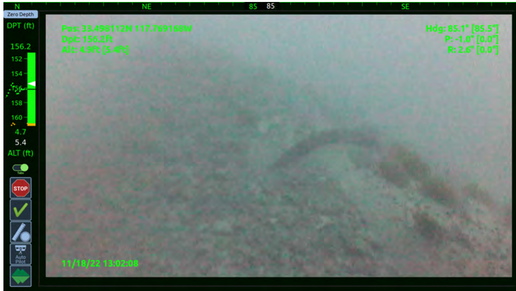
Photo 7 – View showing a section of the ACOO buried by sand
