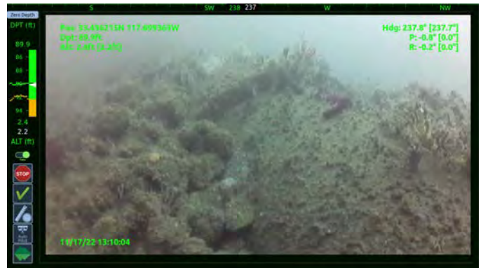
Entry 220 - Flange 21 90% buried
