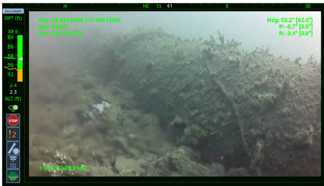
Photo 6 – View of an additional SJCOO diffuser port, with effluent flowing
