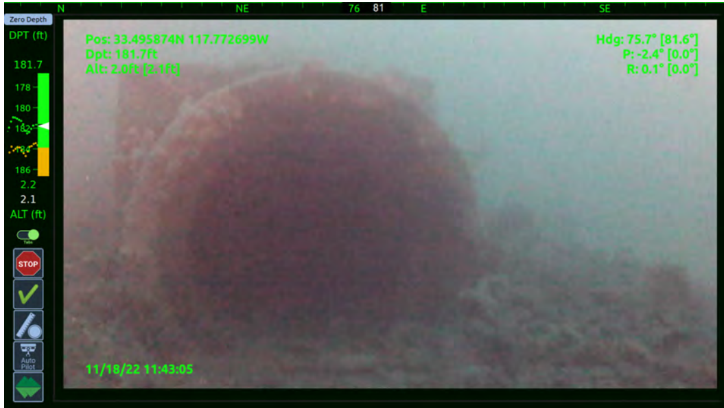
Photo 1 – View at the ACOO end structure
