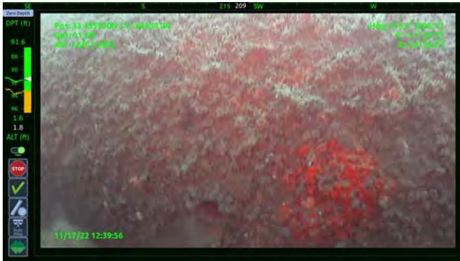
Entry 179 - North side from End Structure D1
