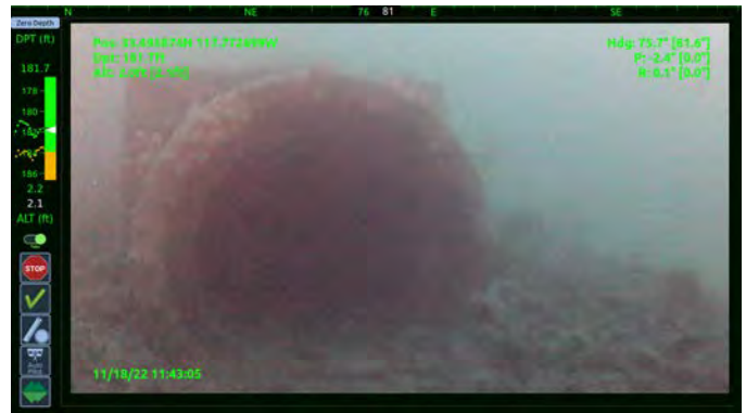
Entry 5 End Structure
