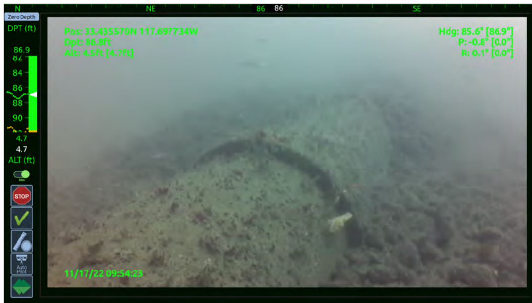
Photo 4 – View showing ballasting covering the top of the SJCOO
