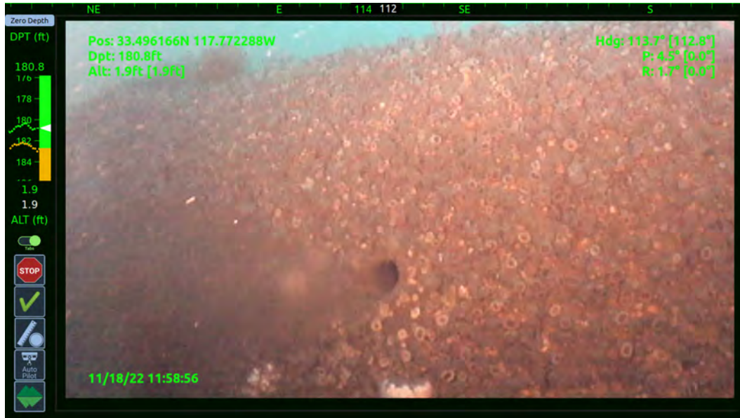
Photo 5 – View of one of the ACOO diffuser ports, with effluent flowing
