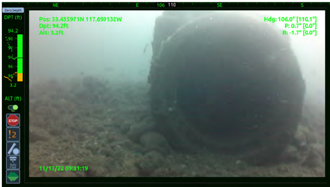
Photo 10 – View of the SJCOO end structure
