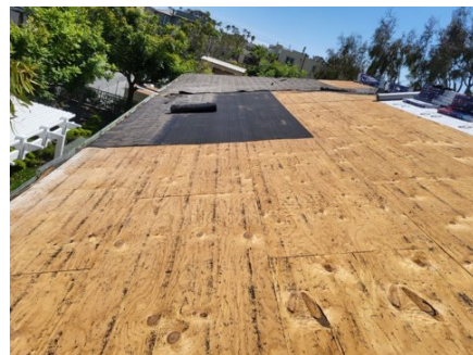
Photo of roofing installation
