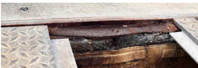
Figure 1. Primary Sedimentation Tank with T-lock Lined Interior
