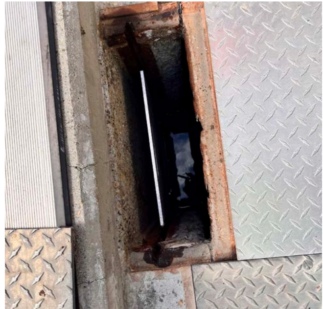
Figure 3. Slide plates are challenging to seat, especially in corroded slots. Replacing plates with manually operated slide gates eases operability of the system.
