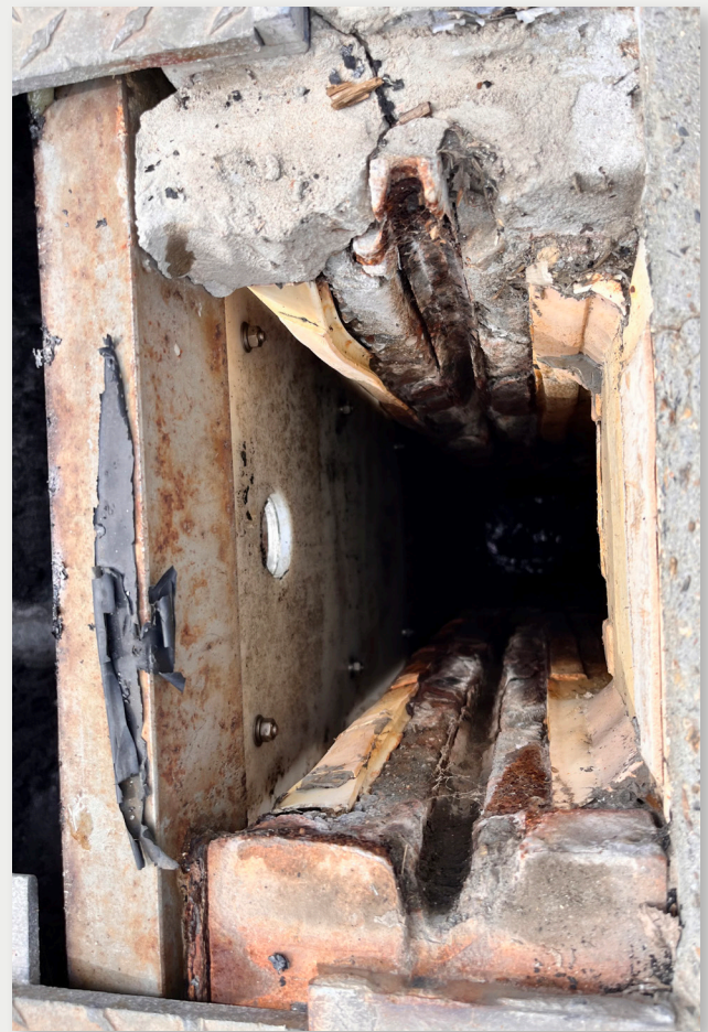
Figure 2. Primary Sedimentation Tank Slide Plate
