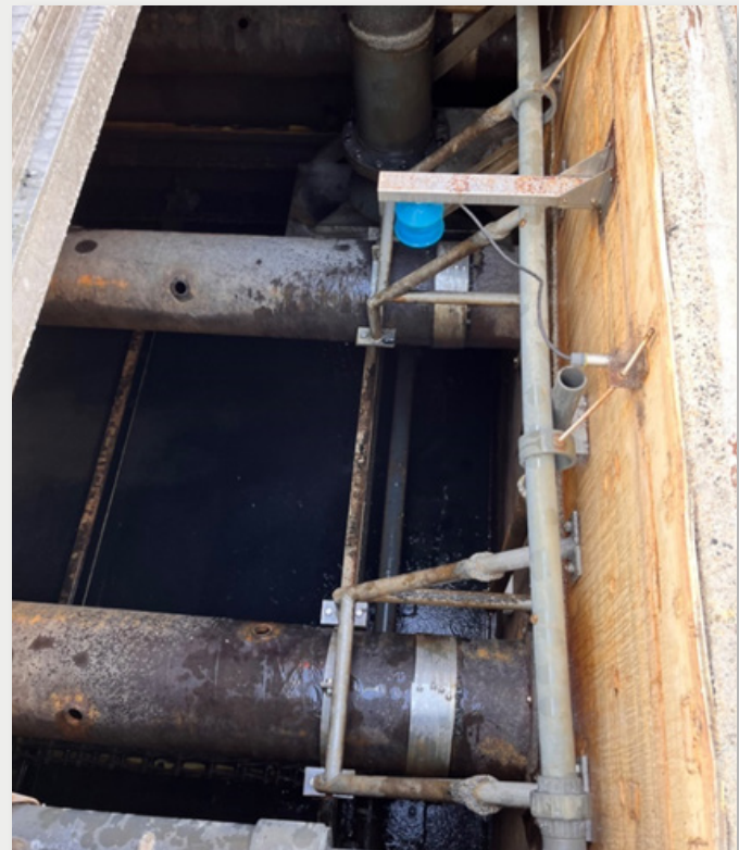
Figure 4. Primary Sedimentation Tank Effluent Pipes
