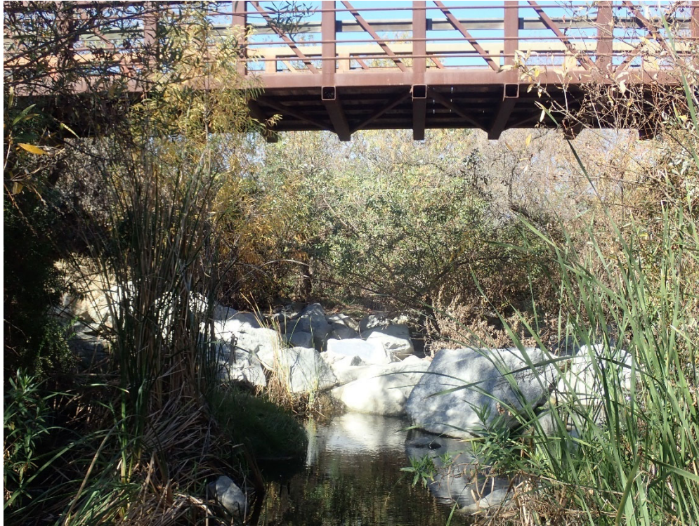
Figure 2.5 – Existing Drop Structure
