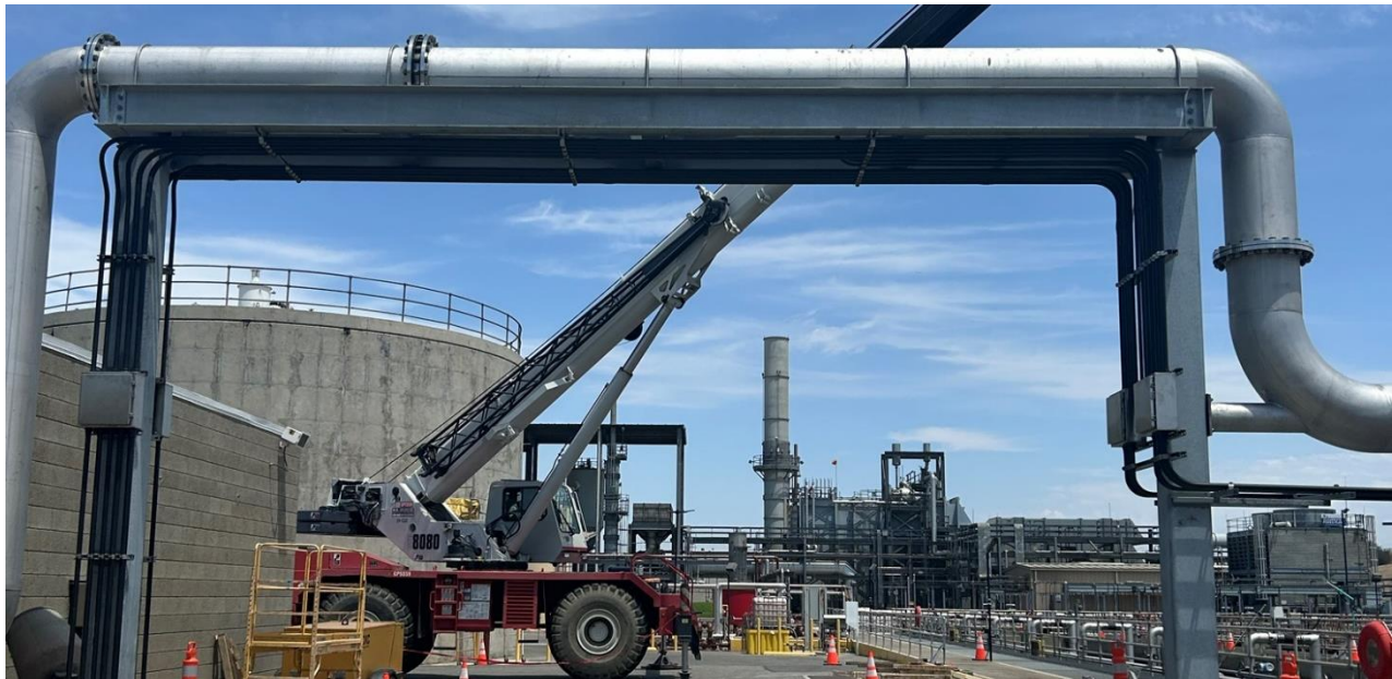
Figure 1. Pipe Bridge Installed for the City of Corona Water Reclamation Facility (WRF) 1A
