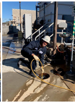
Clearing Drains
