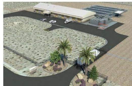
AECOM prepared a master site plan for the ultimate build-out of the site as a 20-mgd Membrane Bioreactor (MBR) wastewater treatment plant. A phased conceptual plan was developed for the WRF to address the initial projected flows up to 3 mgd.
