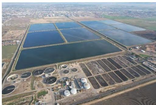
The City currently operates two treatment facilities. Wastewater Treatment Plant No. 2, a 25-mgd trickling filter plant producing secondary effluent stored in dams for agricultural irrigation. Solids are processed through anaerobic digesters and drying beds, yielding Class B biosolids applied to City-owned farmland. Current influent flow is approximately 12-mgd.
