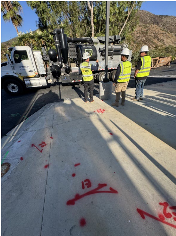
CTP Contractor Potholing Scrubber Area
