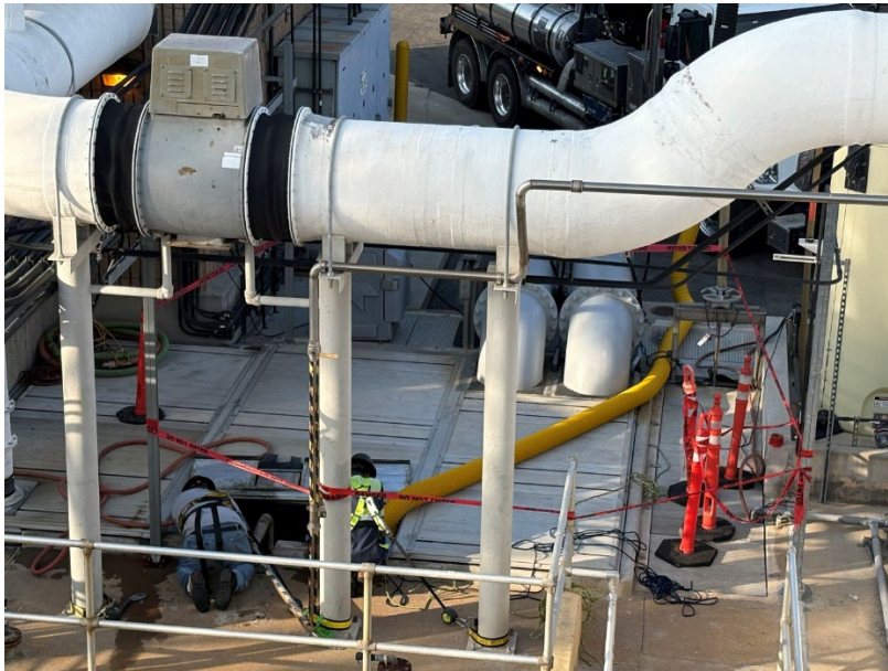
JBL Plant #1 Grit Tank Vactoring
