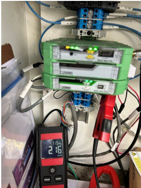
JBL Doheny Outfall Pressure Transmitter Repair
