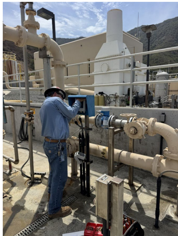
CTP Installation of EQ Flowmeter
