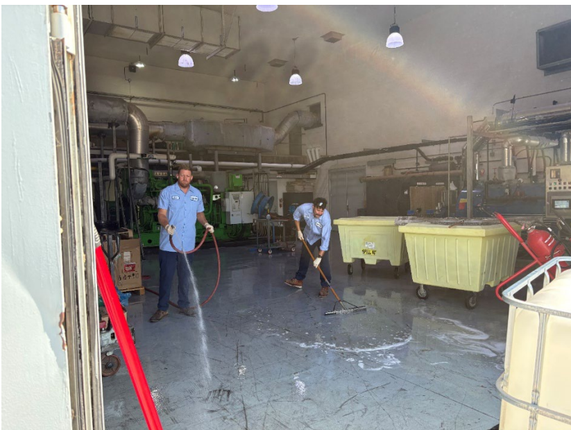
JBL Cleaning Cogeneration Engine Room
