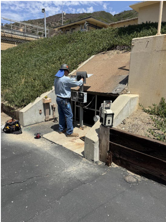
CTP Doghouse Flowmeter Installation
