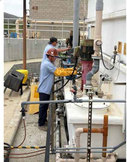
CTP Scrubber Bleach And Caustic Pump Repairs
