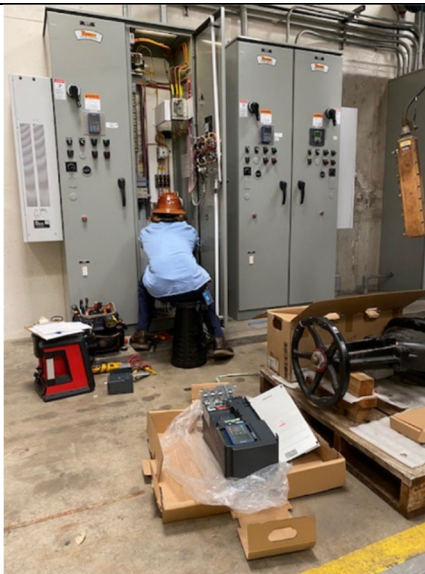
4-Side RAS VFD Replacement
