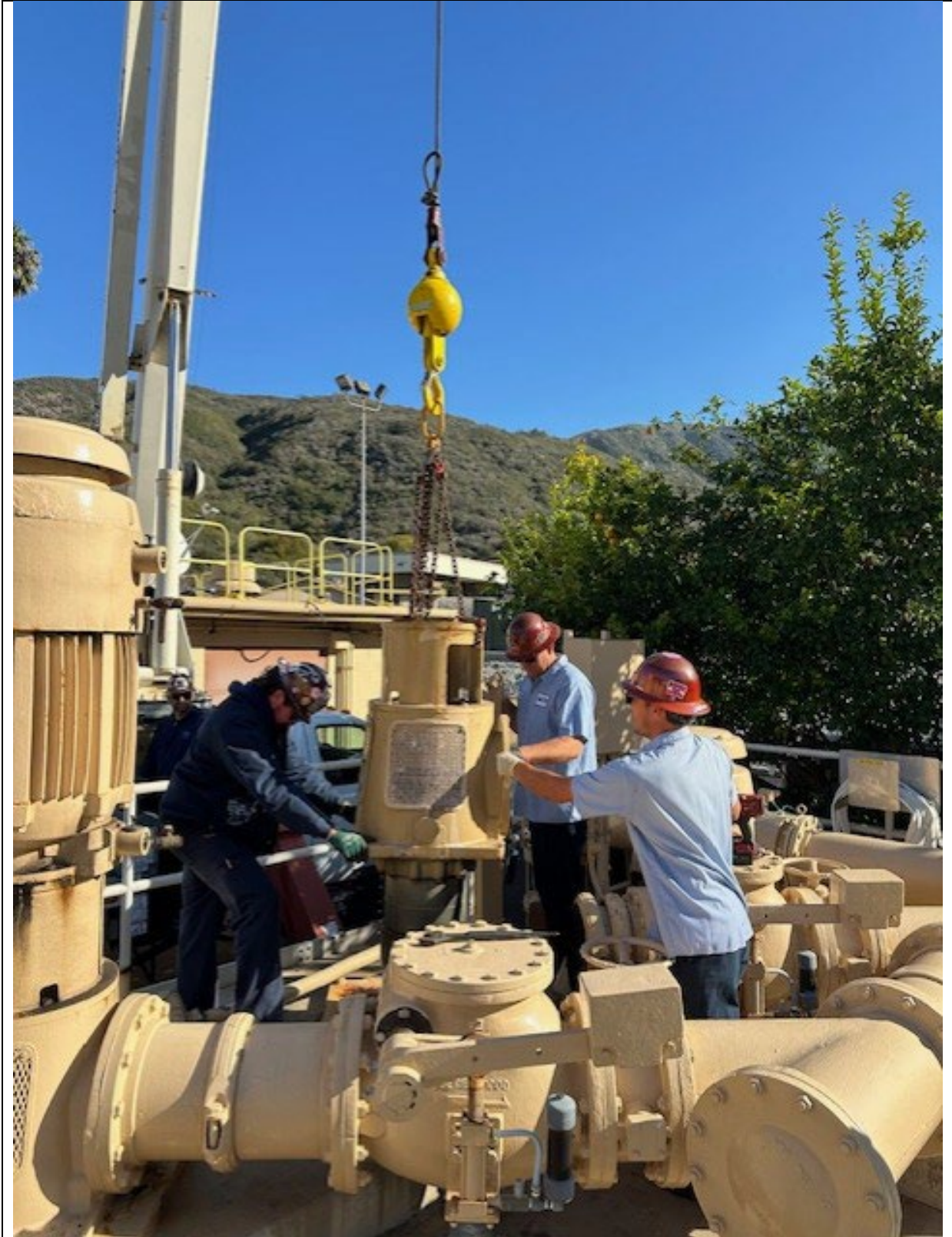
Craning out clearwell #1 pump.
