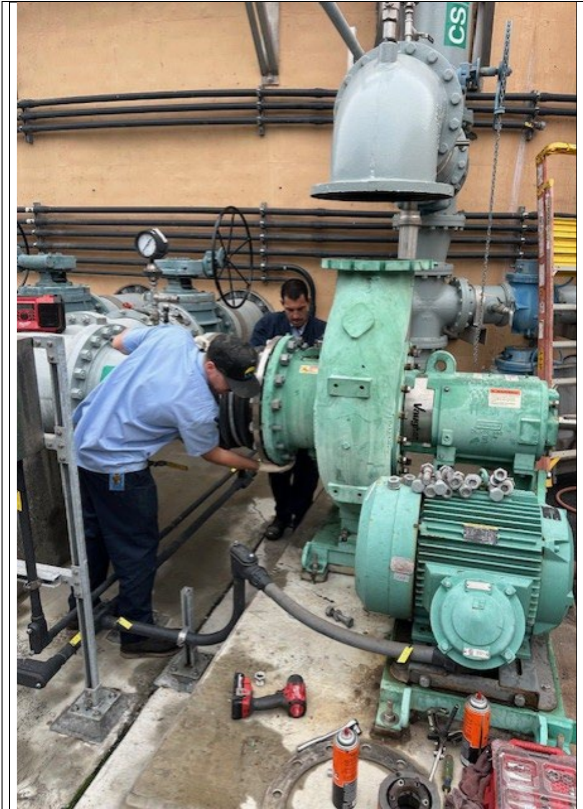
Replacing digester #2 mix pump.
