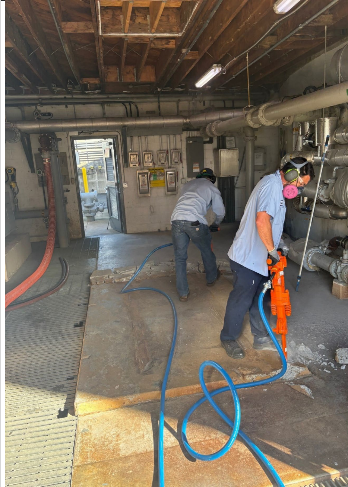
Demo old boiler concrete pad.
