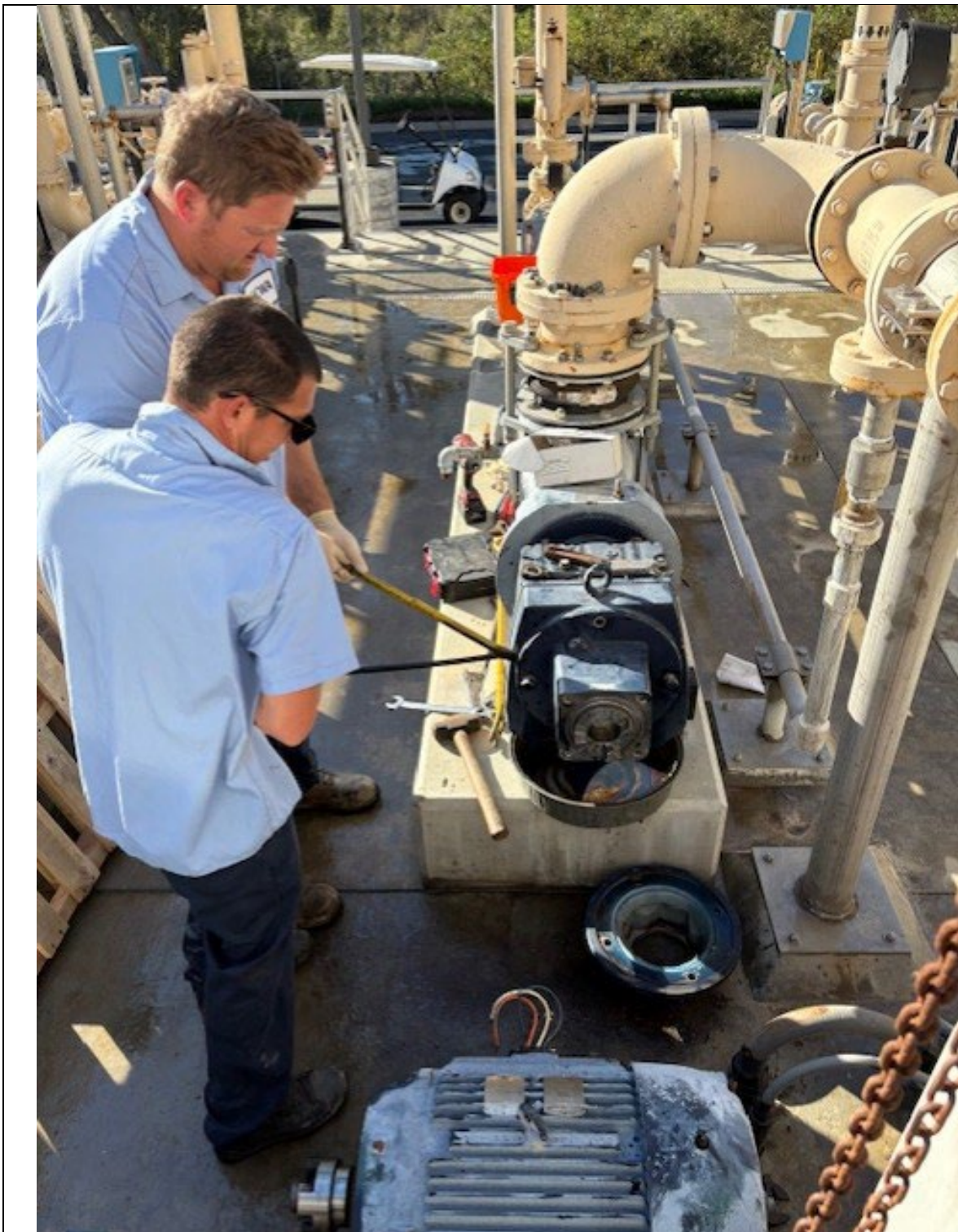
Replacing seal in export pump gearbox.
