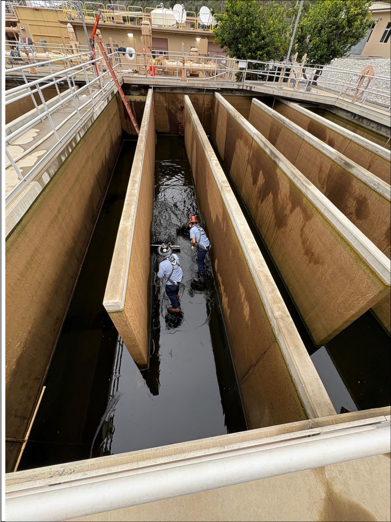
Cleaning contact tank.
