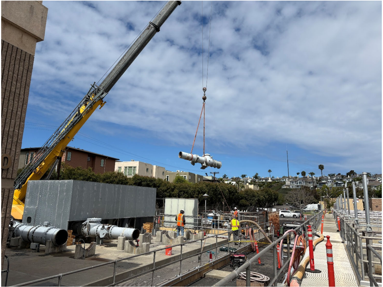
Effluent Pump Station Manifold Replacement
