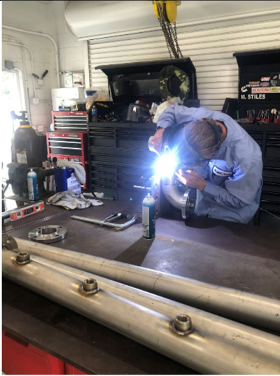
CTP Grit Tank Diffuser Fabrication
