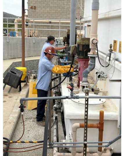
CTP Scrubber Bleach And Caustic Pump Repairs
