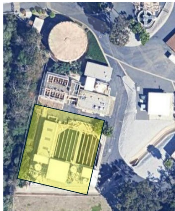
Exhibit 8 -General area - currently occupied by tertiary filters, chlorine contact tanks, and RO - available for a future AWT.
