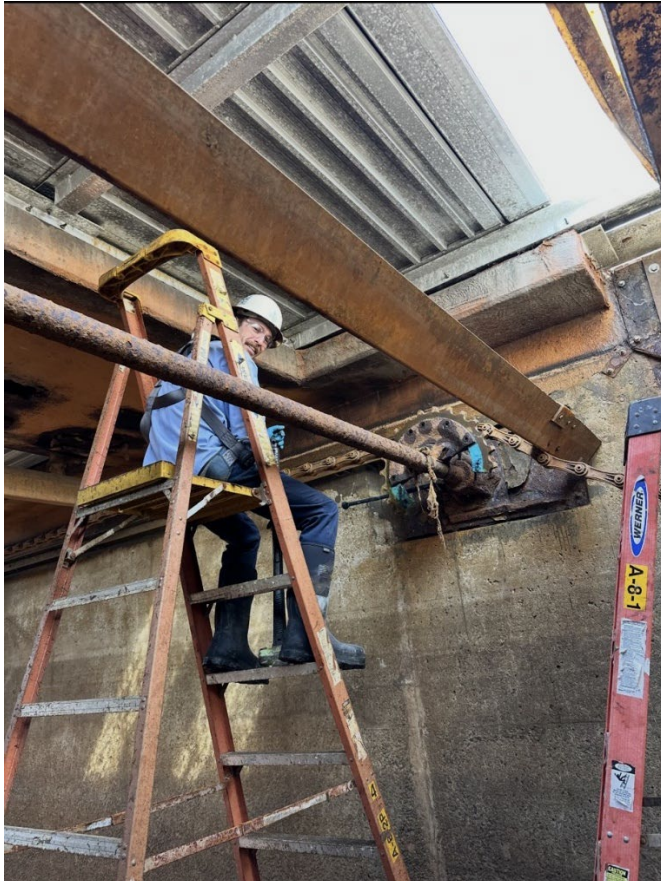
JBL PRIMARY CLARIFIER SPROCKET REBUILD
