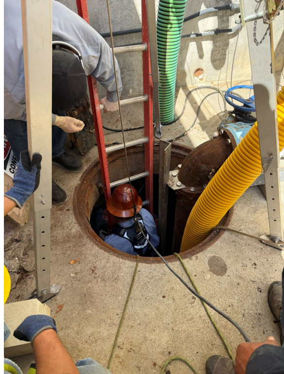
CTP DPS WETWELL CLEANING
