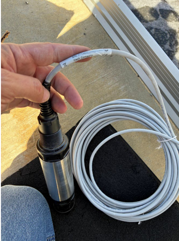
CTP DO PROBE INSTALLATION AND HARDWARE REPLACEMENT
