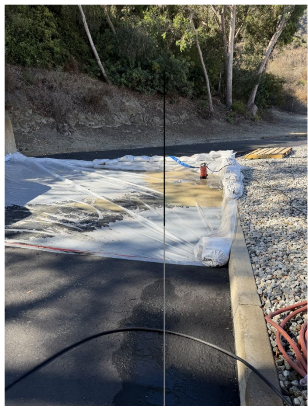
CTP BUILDING #9 PAINTING CONTAINMENT
