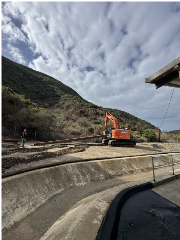
CTP CONTRACTOR STORM DRAIN WORK
