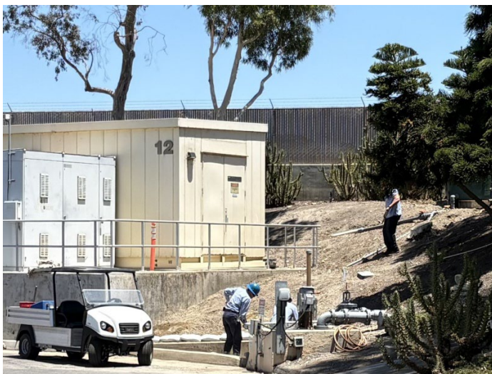
JBL Cleaning Hillside and Plant Sump
