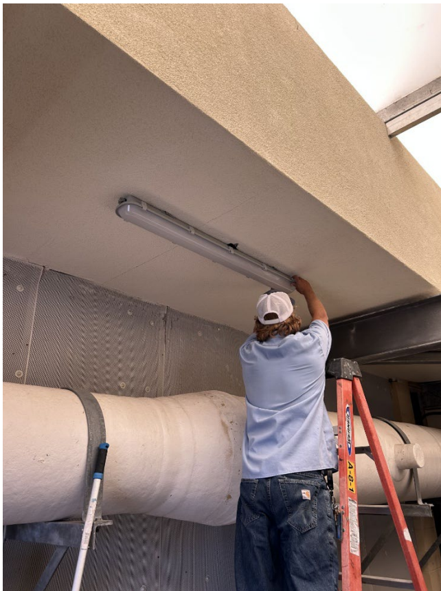
JBL Centrifuge Room Lighting Replacement
