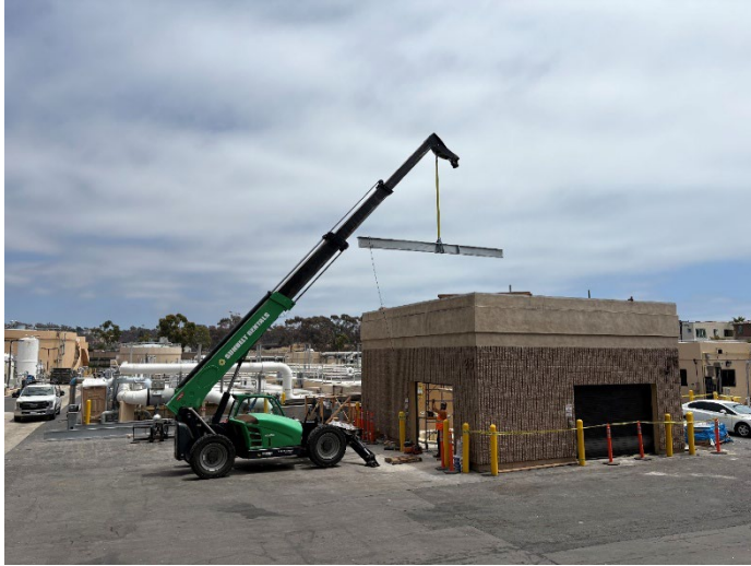
JBL Building #25 Roof Installation
