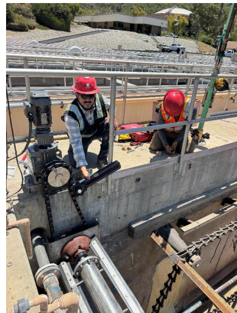
CTP Scum Skimmer Drive Installation
