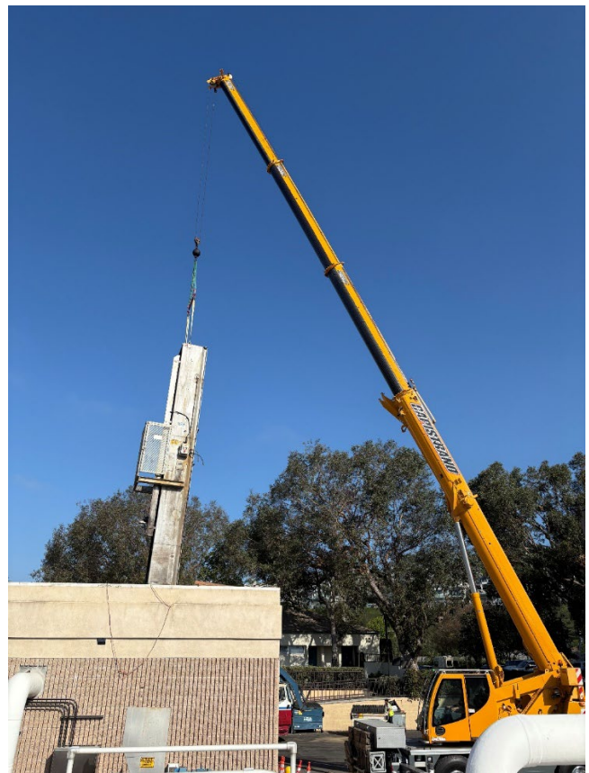
JBL Plant #2 Headworks Barscreen Installation
