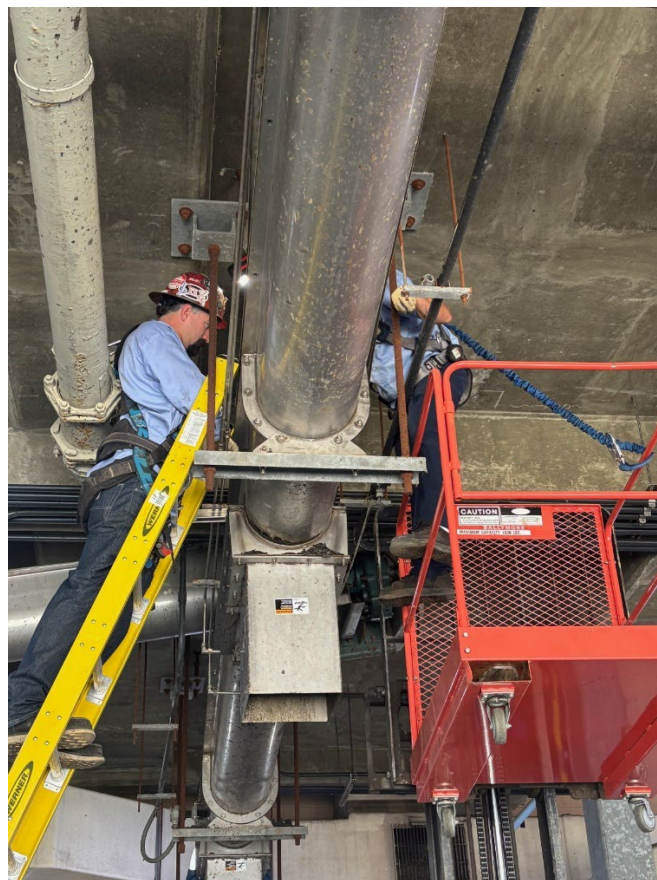
JBL Conveyor Hanger Bearing Replacement
