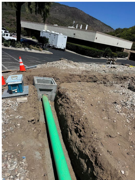
CTP Storm Drain Replacement
