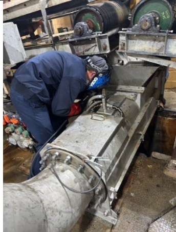
9-Side Vulcan wash press repair
