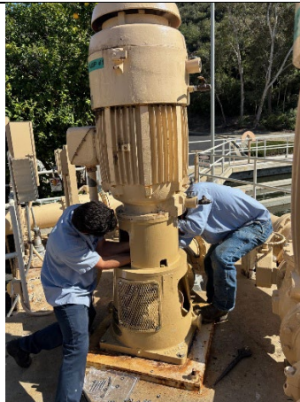
Clearwell pump replacement
