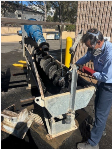
Grit conveyor repair
