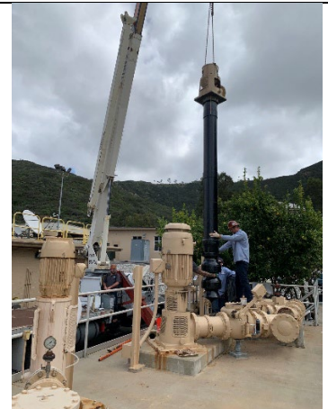
Clearwell pump replacement
