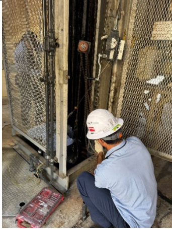
4-Side Bar rake repair
