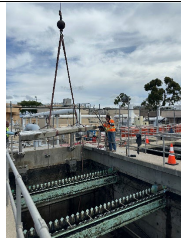
Secondary tank bridge
